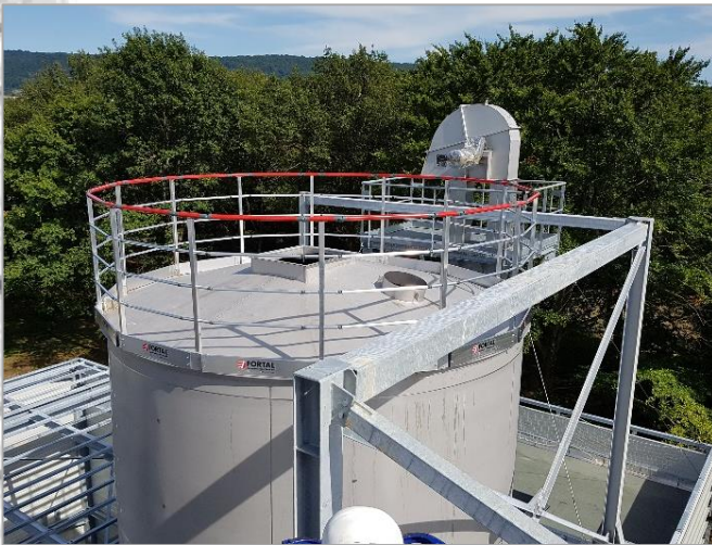
Closer view on fixed guardrails at the top of tank
