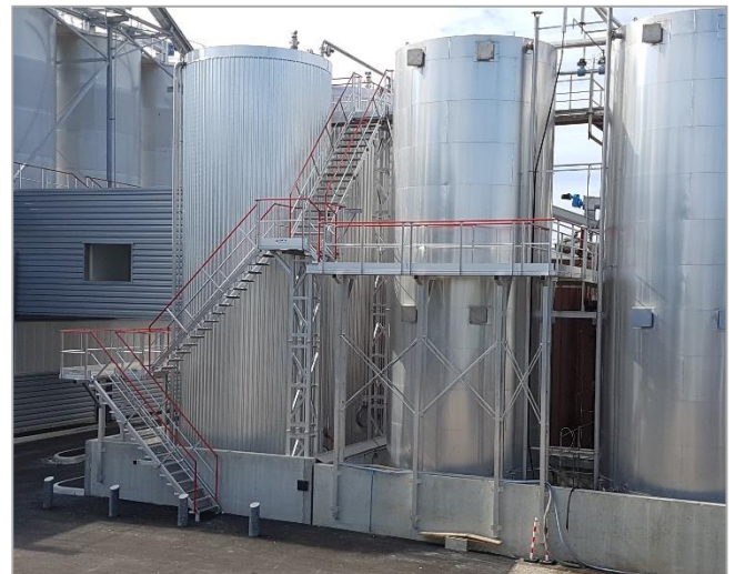
Platforms and gangways represent more than 70 meters length.
