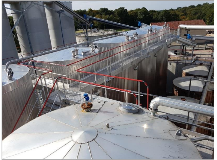
After installation of staircases and gangways for access and pathway.
