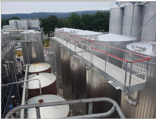
Platforms and gangways represent more than 70 meters length.
