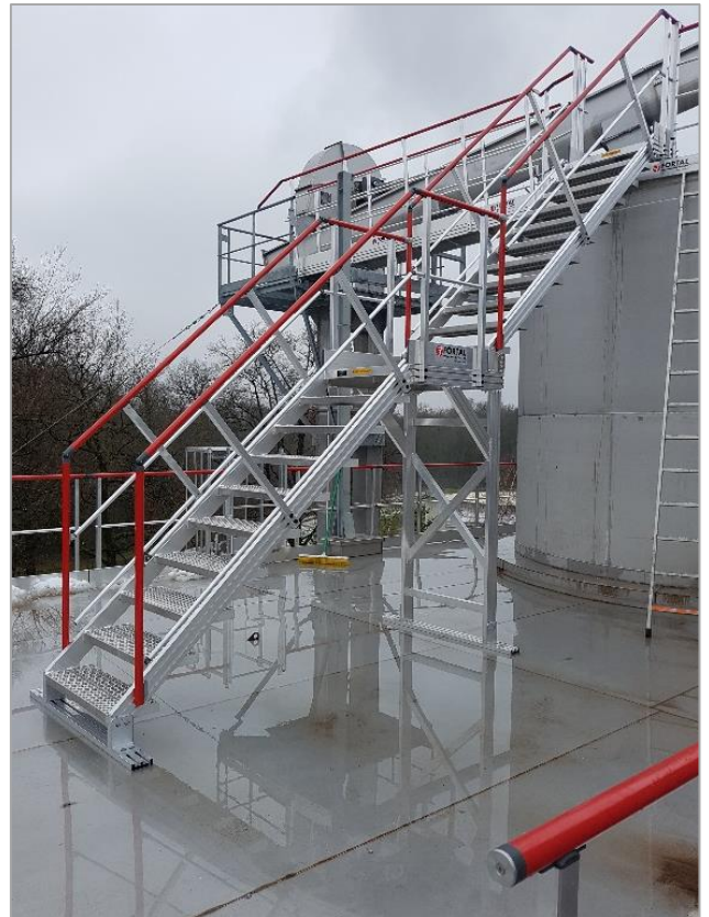
Staircase with platform – grating steps – direct access on the tank.
