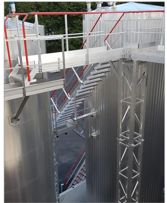
Platforms and gangways represent more than 70 meters length.
