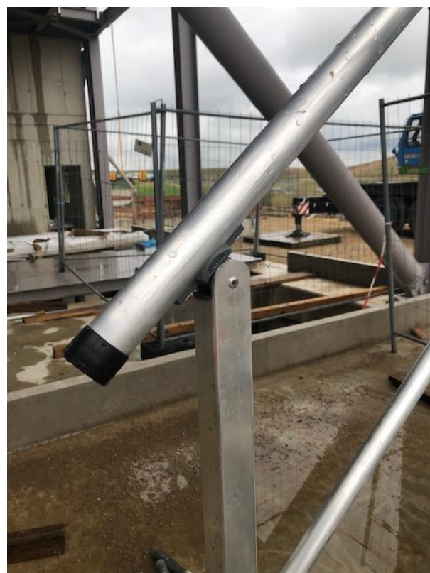
View on poles and handrail
