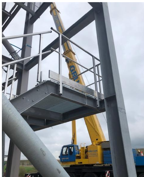
View on poles which make the link between platform and guardrail.
