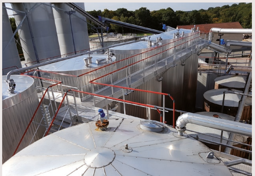
Gangways on storage silos - © FORTAL
