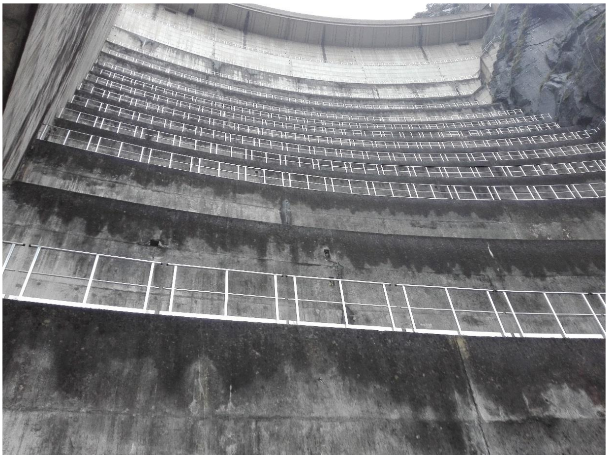
The Monteynard dam, located on the Drac river (France), is 135 meters high and 230 meters width. Its hold 275 million m 3 of water.
