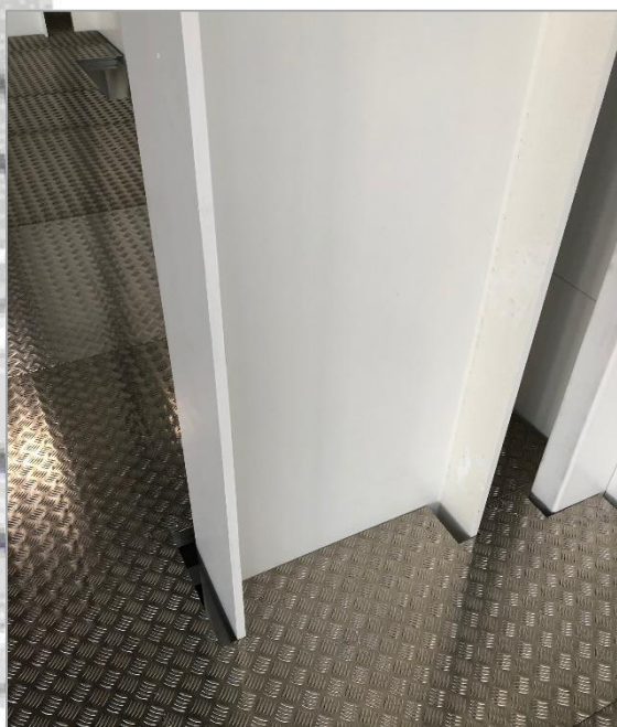
Perfect cut of flat sheet during mounting by the installation team.
