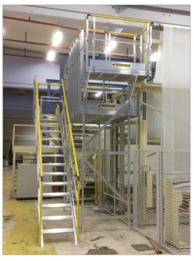
Staircase useful width: 600 mm – anti-slip ribbed aluminum steps depth 261 mm – platform coating: flat sheet aluminum thickness 4.4 mm - ladder to 3rd platform access – guardrail with handrail, intermediary rail and baseboard at platform rear.
