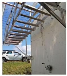
Staircase composed of two parts. The lower staircase can be lifted thanks to a manual winch to allow the movement of vehicles. The upper staircase and the platform are fixed.
