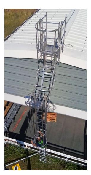
Safety cage ladder for access to the roof of cable car cabins station. Due to the shape of the hosting structure, the ladder is composed of three parts.
