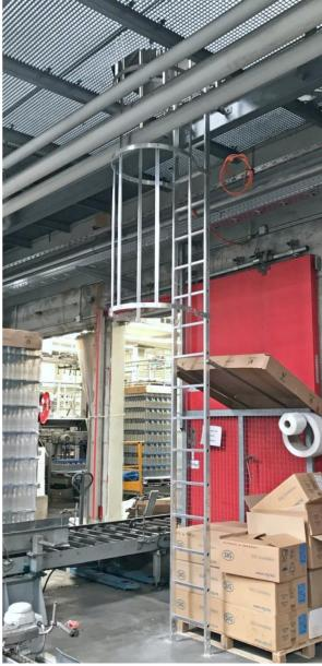
Aluminum profile 65 x 25 mm safety cage ladder for access to the upper floor.
