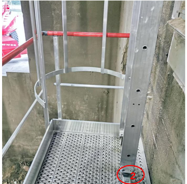
View on the low part of the « mobile » safety cage ladder
