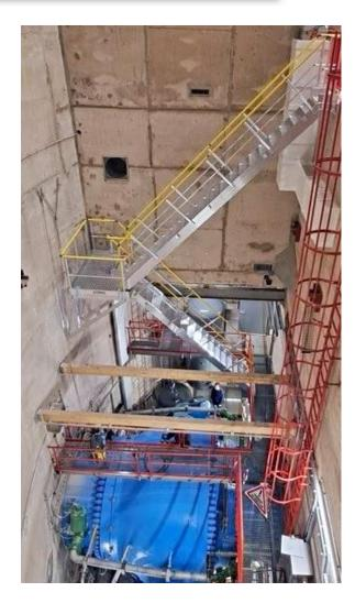
Staircase with landing platform in extruded raw aluminum profile 100 x 30 mm for emergency evacuation of the turbine area – total height 9250 mm. Aluminum 6000 series offering high corrosion resistance and is maintenance free.
